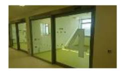
Single sliding door with fixed glazed panel, selfsupported, fitted within door opening
